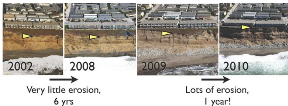
Figure 8.56. Coastal Erosion in Pacifica
